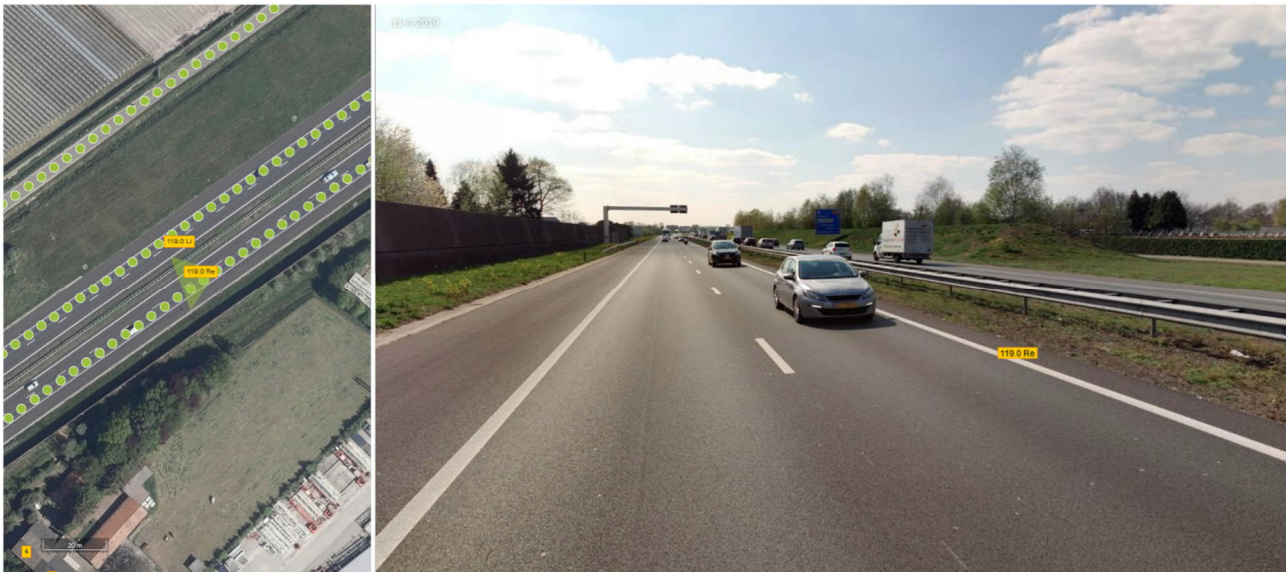
Figure 6.2: Section of the PA 8 with 40% RA in the A50 near Veghel; realized in August 2016; photo from April 2019
